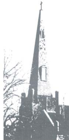
Steeple Preservation Completed November 2009
