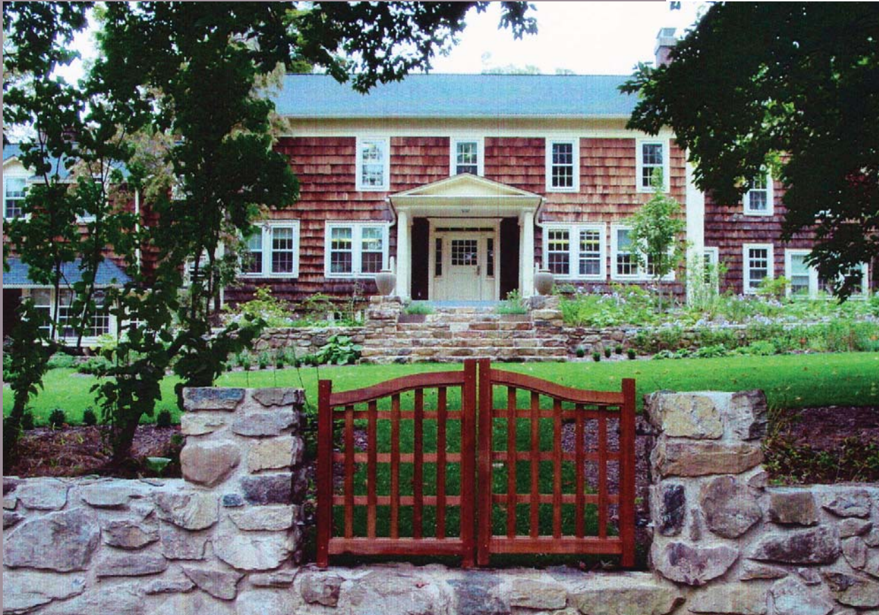
COMPLETED PROJECTS: Bamboo Brook Outdoor Education Center, Morris County (also on the cover). PAGE 8
