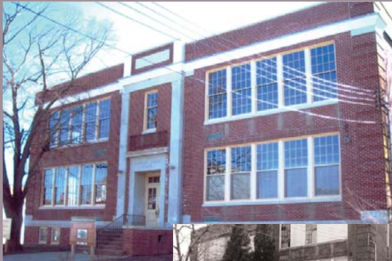
Franklin Street School, after the first phase of rehabilitation
