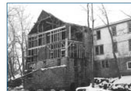
Restoration and stabilization at the Mill continues.
